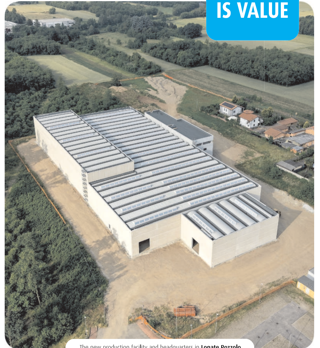
The new production facility and headquarters in Lonate Pozzolo
